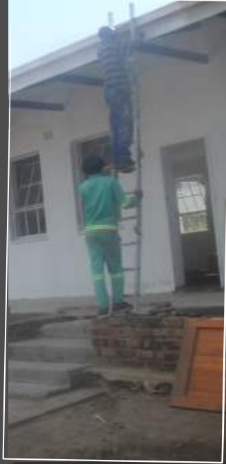
Renovation of Segwelane primary school
