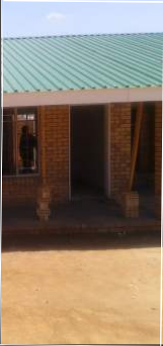
Lekgopung clinic project
